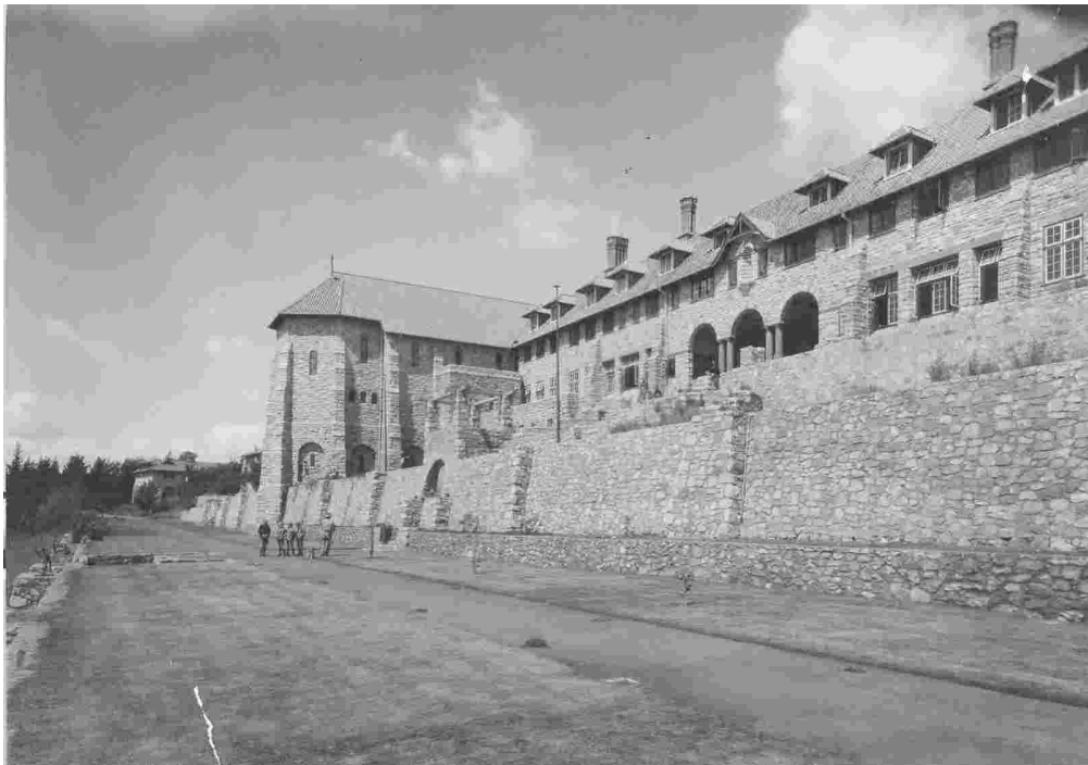
ST JOHN'S COLLEGE, HOUGHTON – BUILT IN 1927 THE NORTH WING SHOWING TERRACES AND THE CHAPEL
